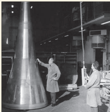
An inner conductor for the new neutrino “horn”.
